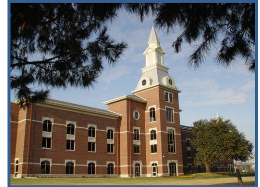
Parking structure built using the Design-Build delivery method for Baylor University.
